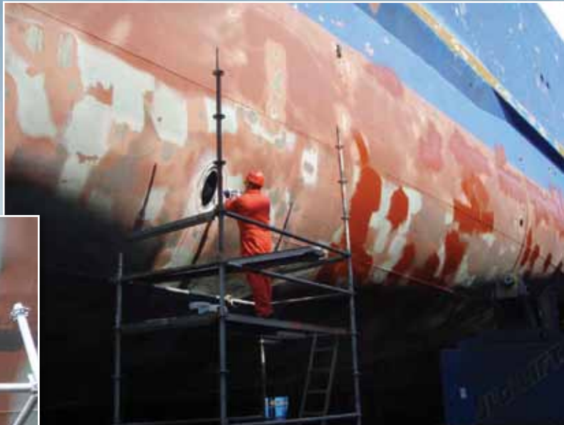
Elliptical anode being fitted
